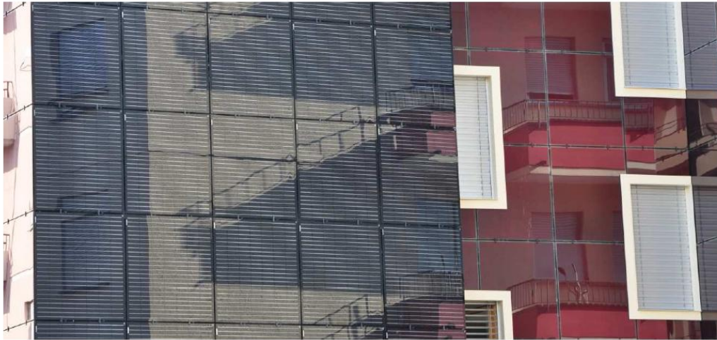
PALAZZO POSITIVO IN CHIASSO (SWITZERLAND), REFURBISHMENT WITH A BIPV COLD FACADE (SOURCE: F. FRONTINI, SUPSI)
